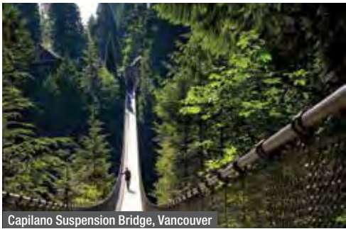
Capilano Suspension Bridge, Vancouver
