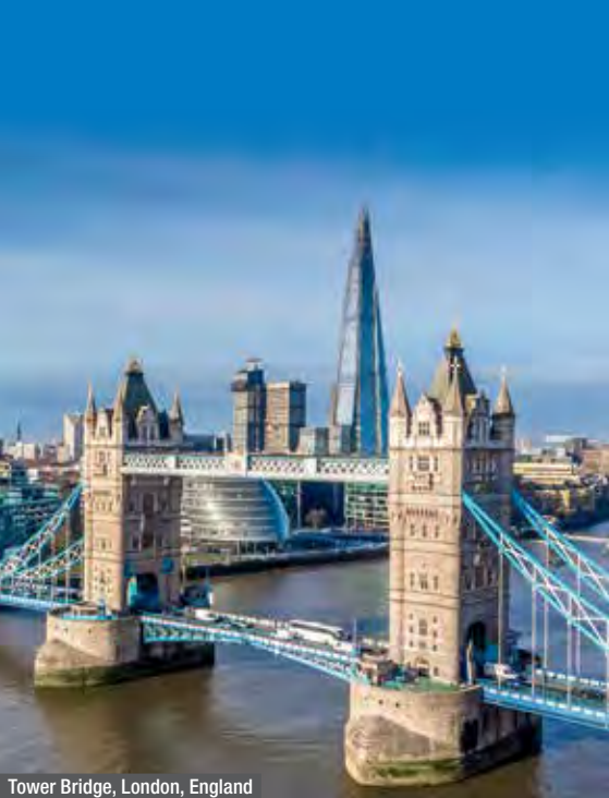
Tower Bridge, London, England
